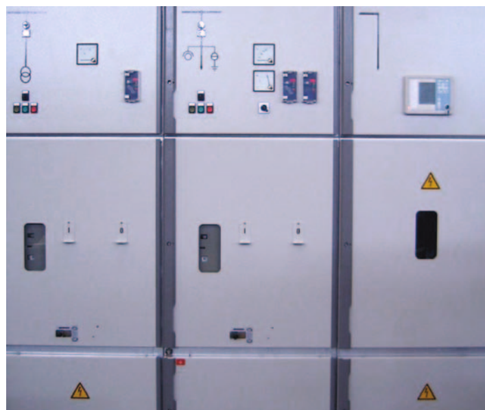
10 kV SPREPOWER medium voltage switchgear
